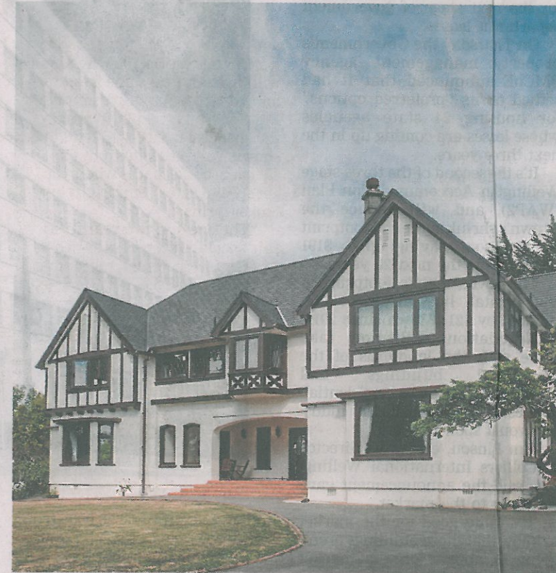
The "ambassador's residence" in Lower Hutt proved to be a much bigger job than first expected.
