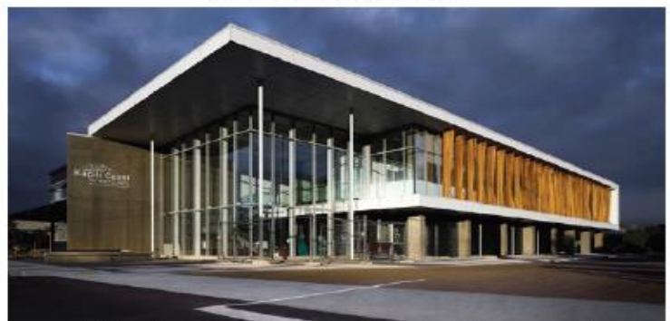
Silver Winner - Armstrong Downes Commercial Kapiti Coast District Council Administration Building
